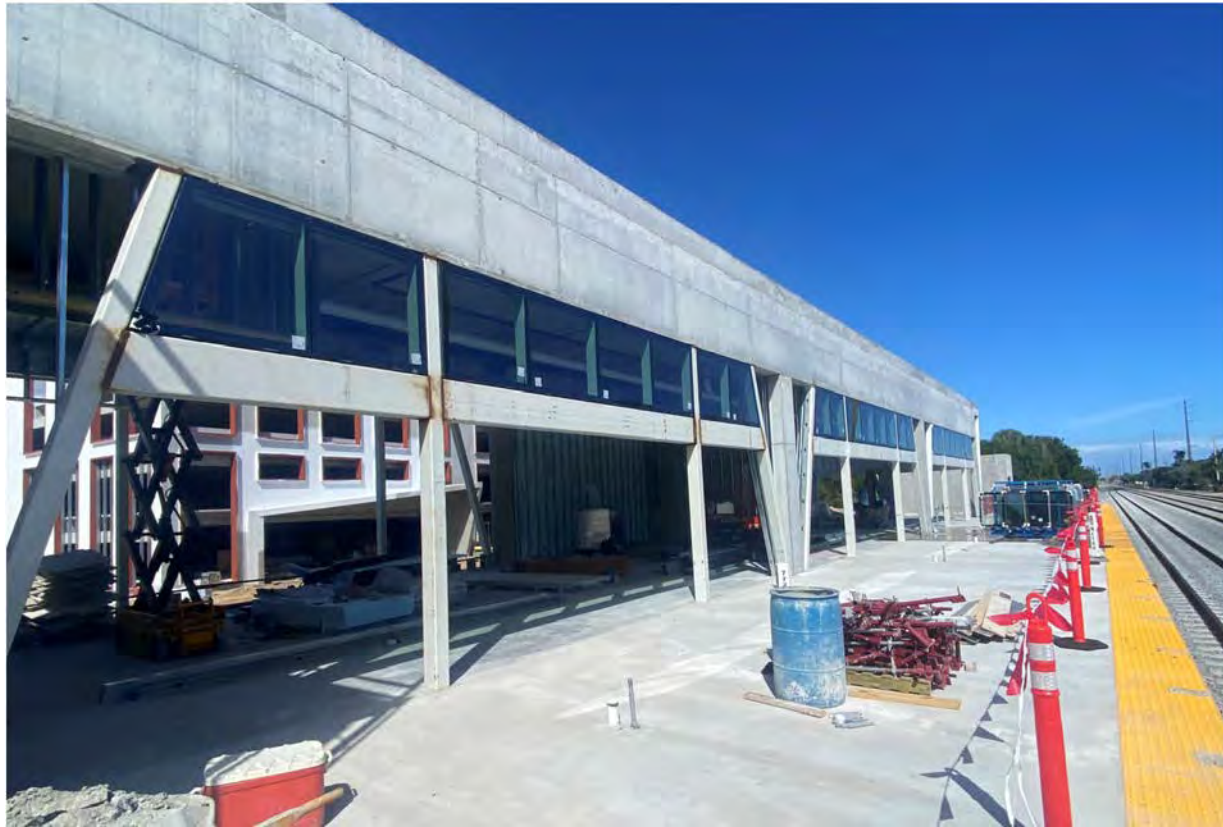
Boca Raton station and platform
